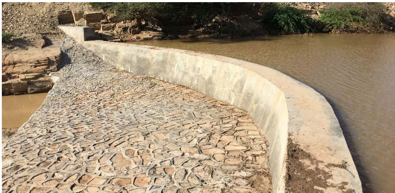
Figure A5 | Sand Dam in Somalia Used as Green Infrastructure for Aquifer Recharge
