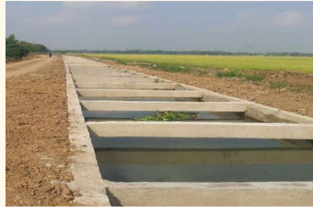
Rehabilitasi SS Kalong
