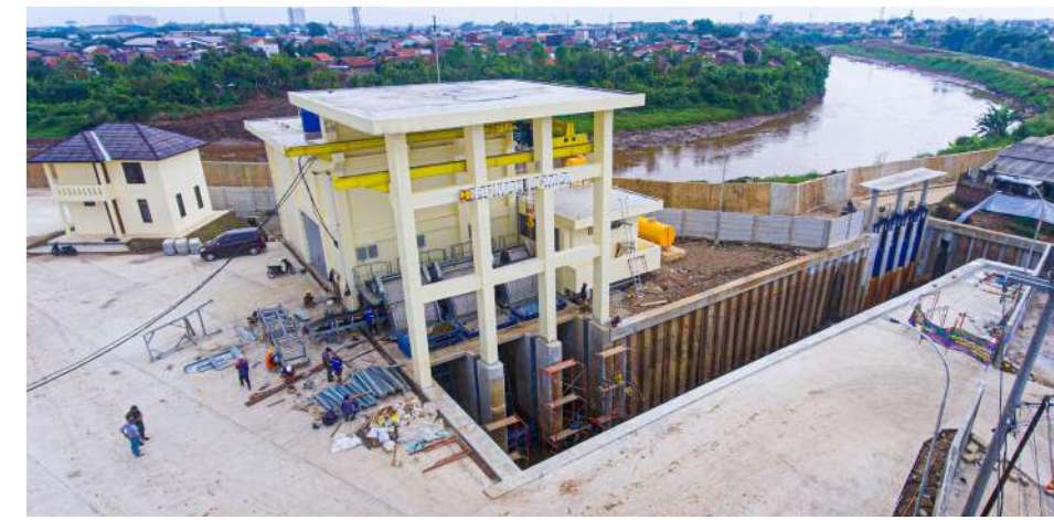
RUMAH POMPA ANDIR (on going)
