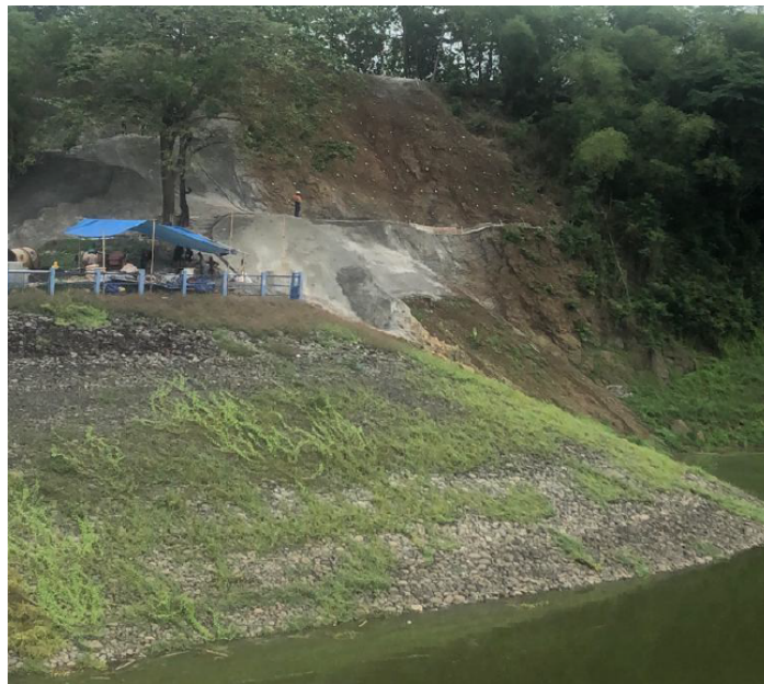
Figure 6-3. Condition Slope on the Upstream Right Abutment (Photo -1)
