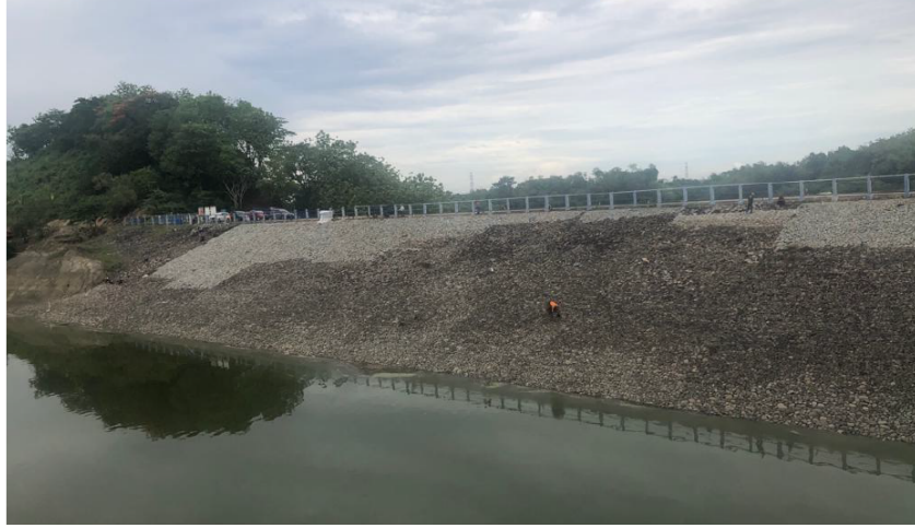
Figure 6-4. Riprap for Slope Protection on the Upstream Dam (Photo -2)
