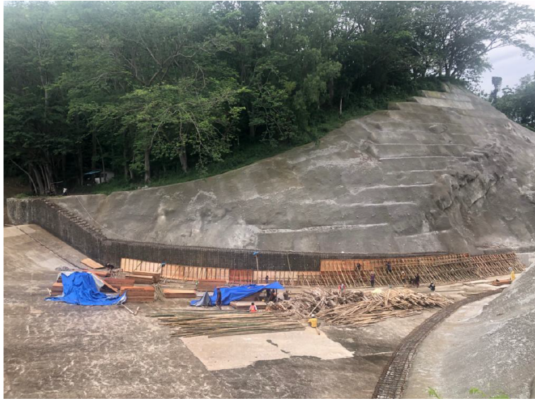
Figure 6-5. Condition of Spillway Left Bank Concreting Works (Photo -3)
