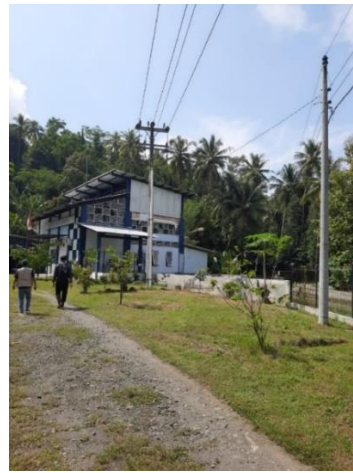
Foto 10. Power House PLTMH Semawung Tampak Samping
