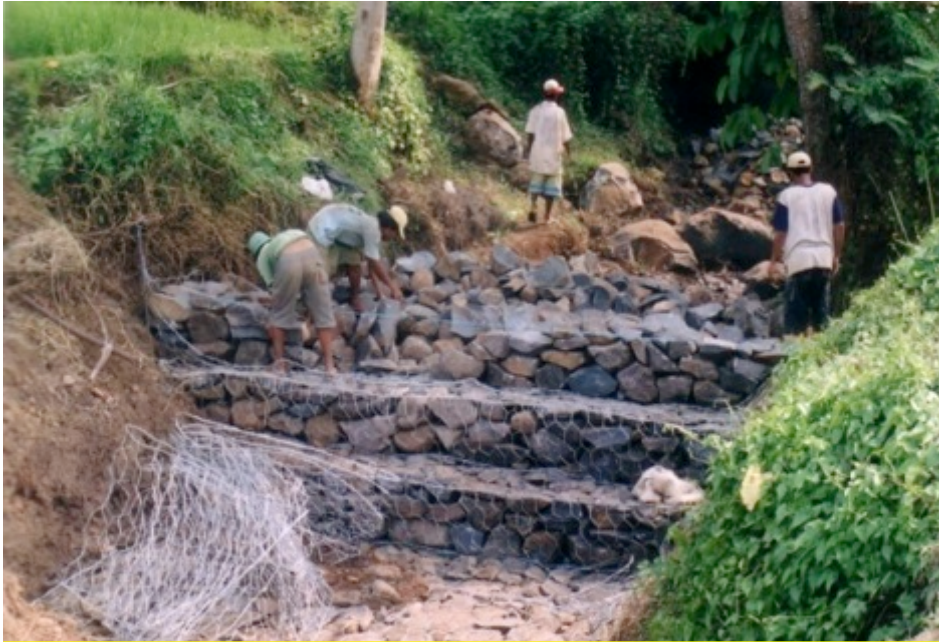
Small checkdams to address overland erosion
