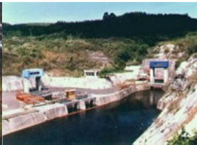
Tulungagung Tunnel (Neyama)
