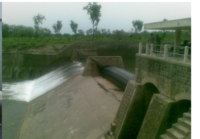
Jati Rubber Dam
