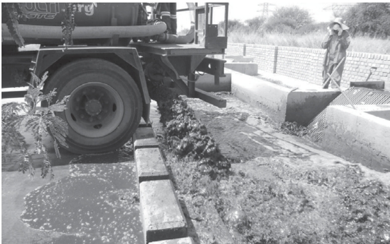
Photo 6.3 Flat apron receiving unit that could be improved by adjusting the levels so that the apron is lower than the road, Gaborone, Botswana
