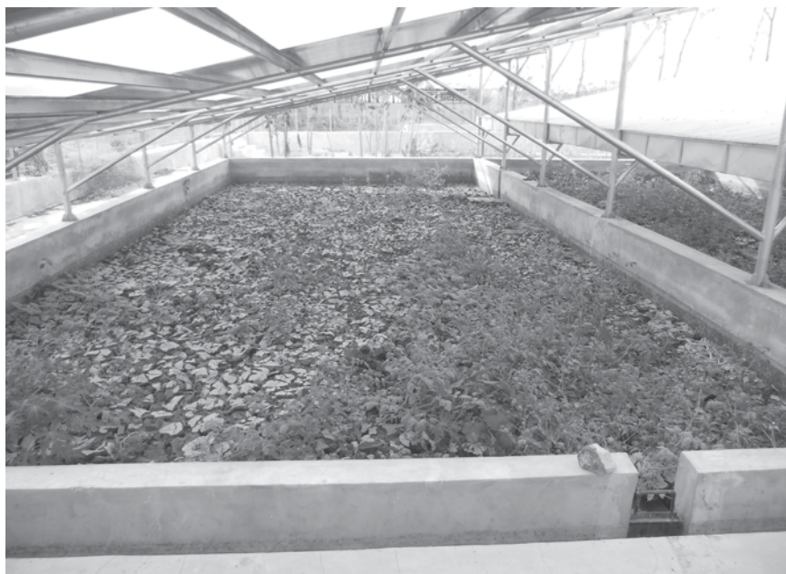
Photo 9.2 Drying bed cover arrangement, Jombang, Indonesia
