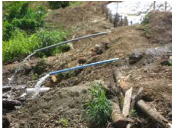
Figure 6. Drainage pipes
