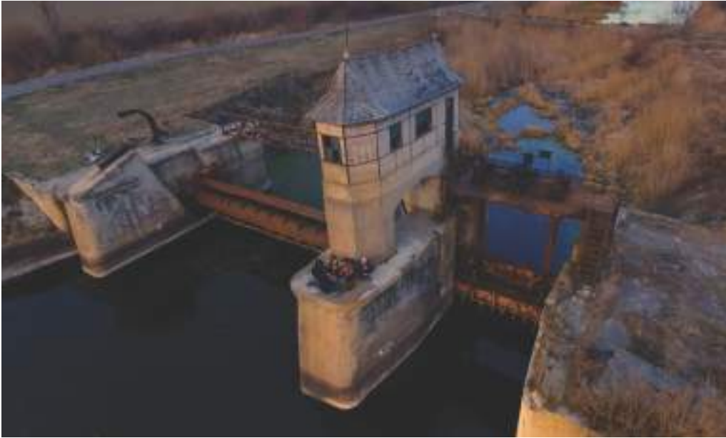
PHOTOGRAPH 3.8. View of the Sanmihaiu Român Dam
