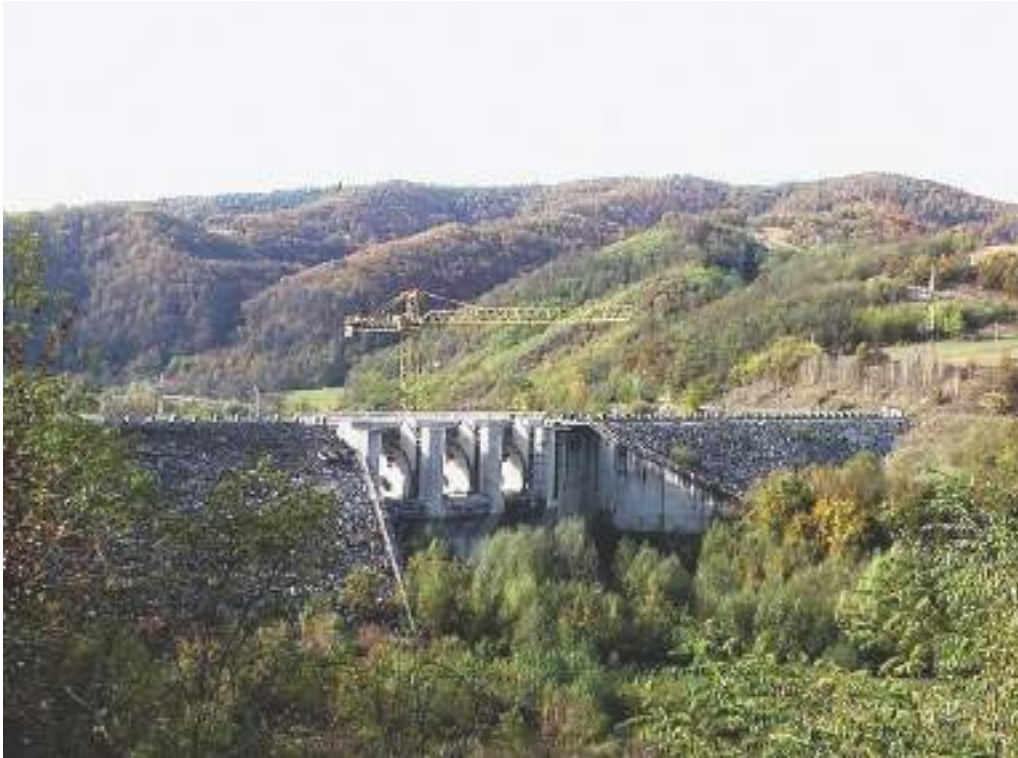
PHOTOGRAPH 3.9. View of the Mihăileni Dam
