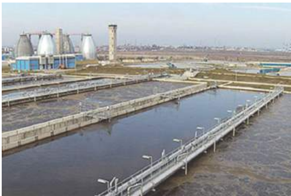
PHOTOGRAPH 7.3. View of the New Bucharest WWTP ( Apa Nova Bucuresti )
