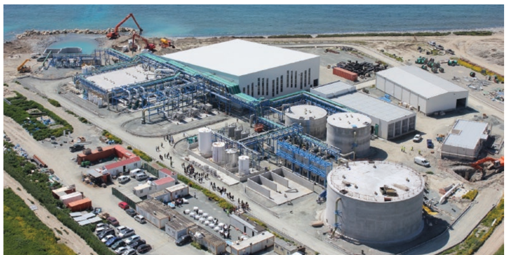
PHOTOGRAPH 2.7. View of the Limassol Desalination Plant
