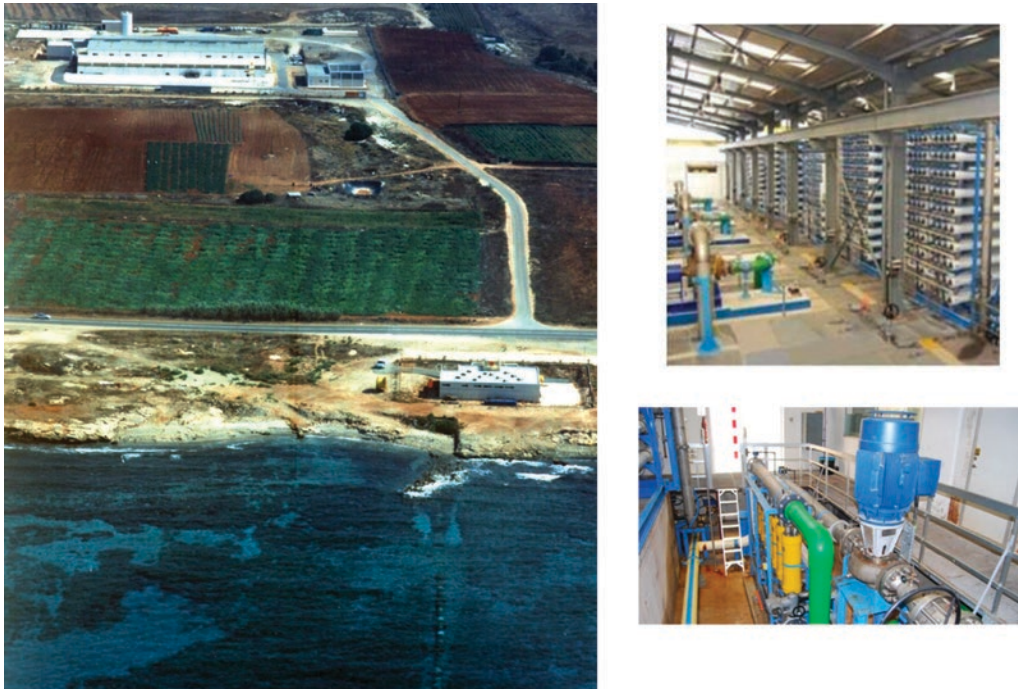
PHOTOGRAPH 2.5. The Dekhelia Desalination Plant
