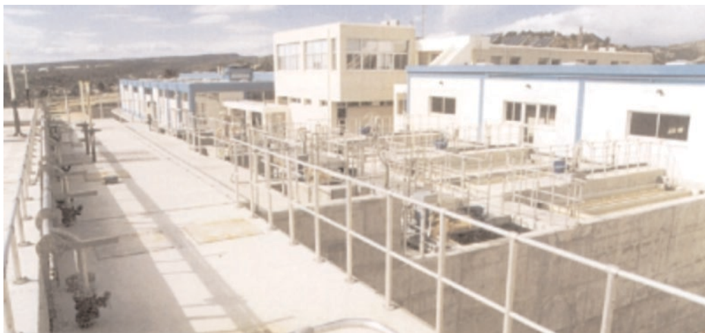
PHOTOGRAPH 2.3. General View of the Limassol Water Treatment Plant
