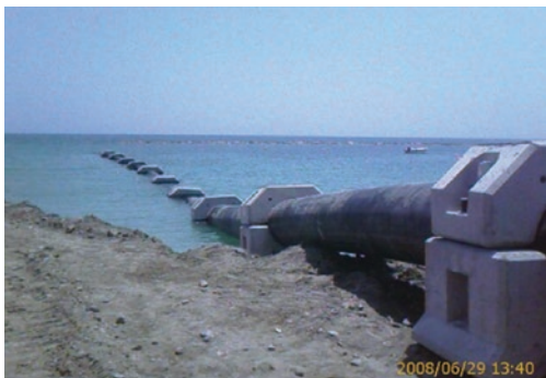
a. Construction of sub-sea supply pumping main
