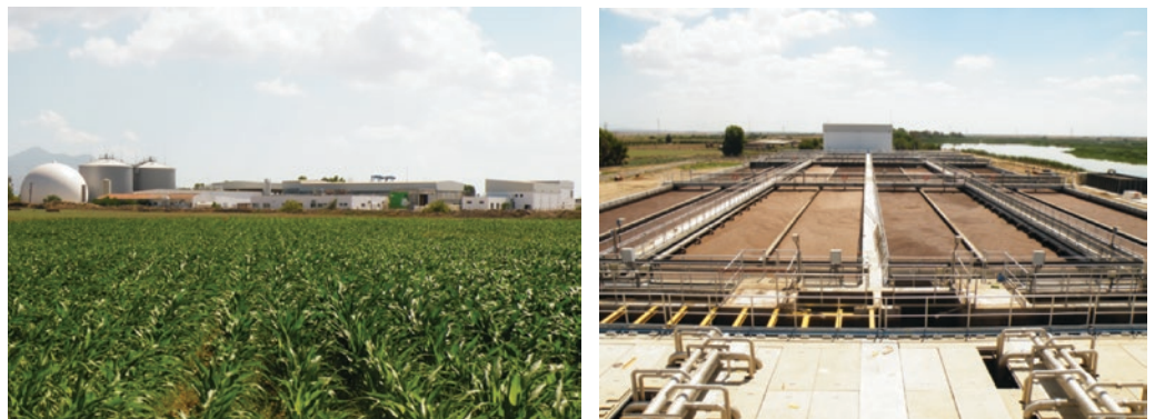
PHOTOGRAPH 2.10. View of the “New Nicosia” Bicommunal WWTP
