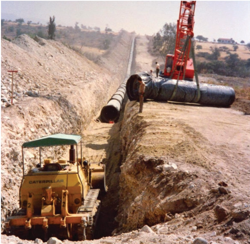
PHOTOGRAPH 2.2. Laying of Main Conveyor's Pipeline
