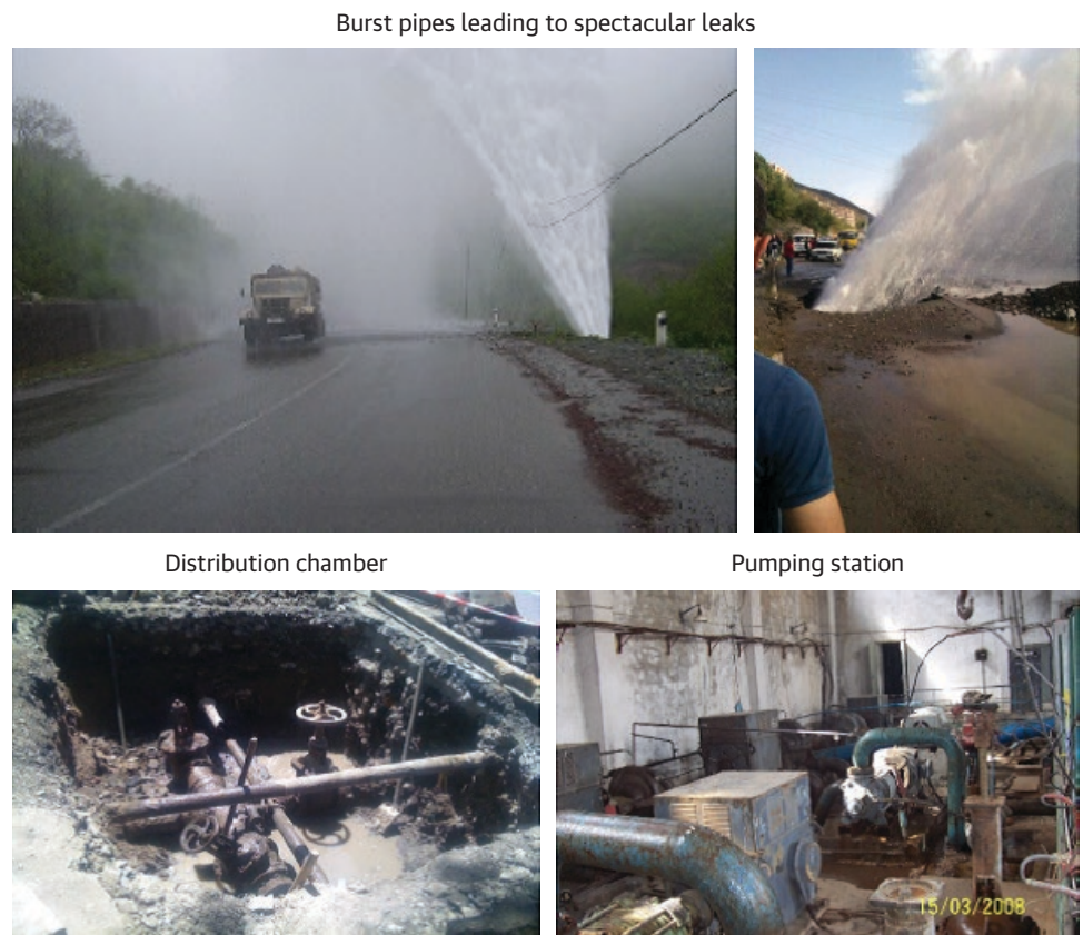
PHOTO 4.1. State of Water Infrastructure before the AWSC Management Contract
