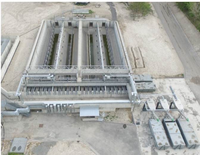
PHOTO 8.1. New Wastewater Treatment Plant in Yerevan
