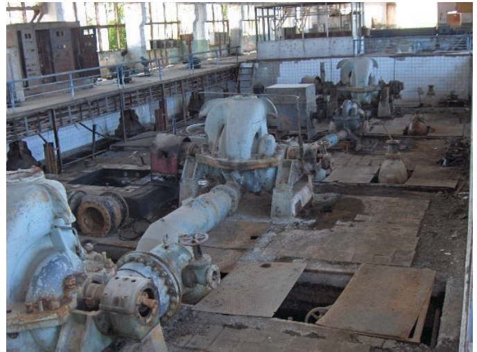
PHOTO 1.1. Masis Pumping Station
