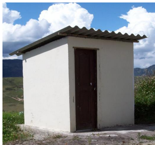
Photo 2-1: Typical Latrine Superstructure, Ecuador
