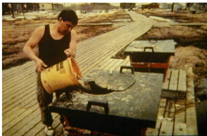
Photo A1-2: Emptying Wastes into Intermediate Tank, Alaska
