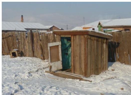
Photo 1-1: Pit Latrine, Ulaanbaatar
