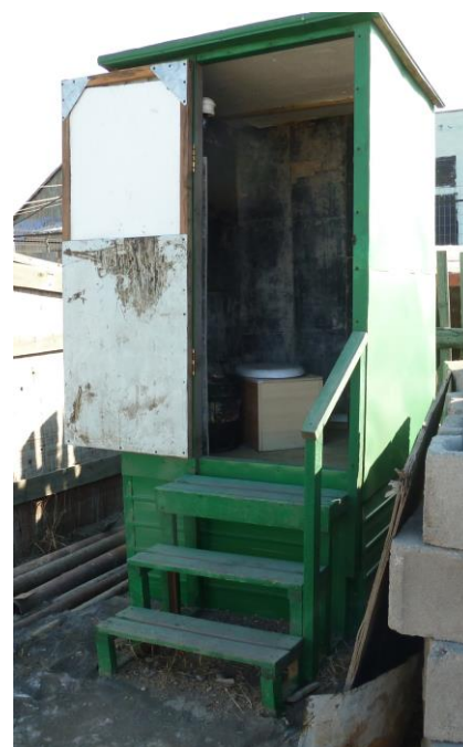
Photo A5-2: Container-based sanitation, household toilet facility, Ulaanbaatar
