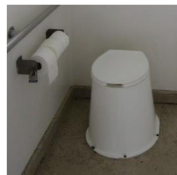
Photo 4-3: Pit latrine with seat and finished floor, Alaska
