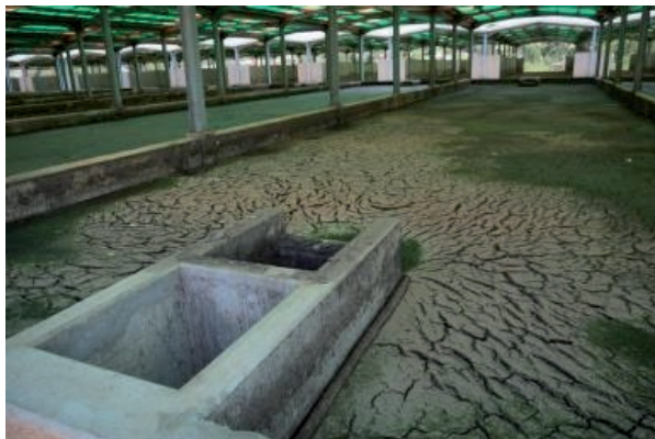
Covered drying beds at the NWSC's Lubigi works, where the NWSC produces compost for sale to market gardeners and farmers.
