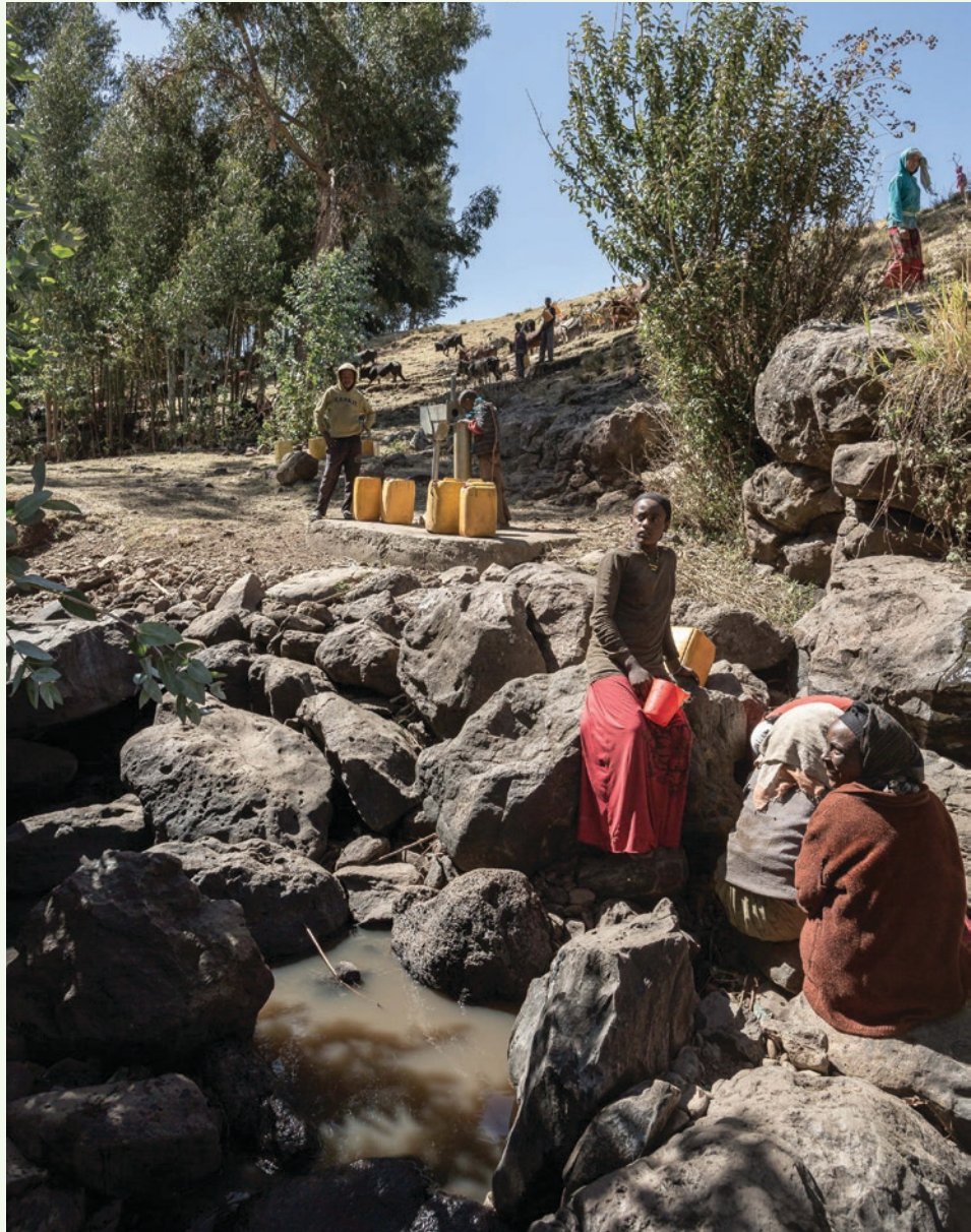
Broken water point in Arsi Woreda Oromia. © Chris Terry/World Bank
