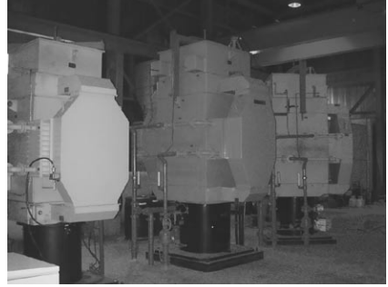
Figure 4: Irrigation district pumps in the Luck Lake Pumpstation.
