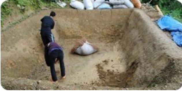
Figure 1. Smoothing of inner wall of Jalkund.
