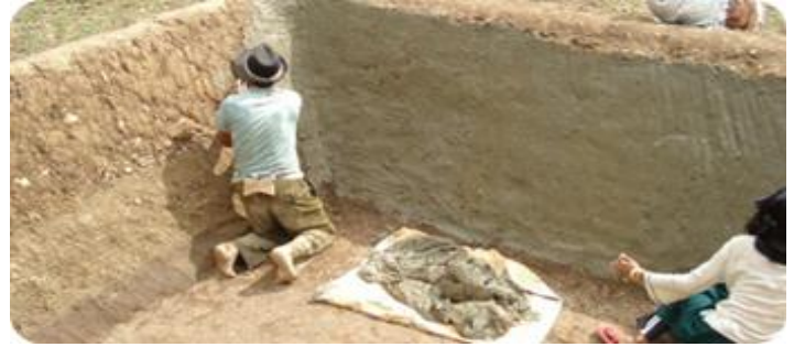
Figure 2. Plastering of inner walls of Jalkund.
