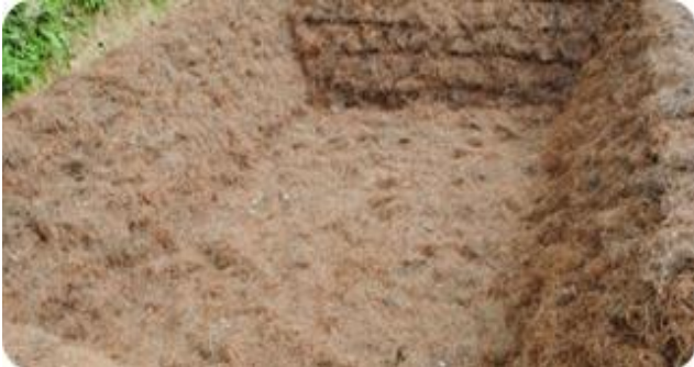
Figure 3. Cushioning of inner walls of Jalkund.
