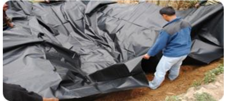
Figure 4. Laying of LDPE for Jalkund.
