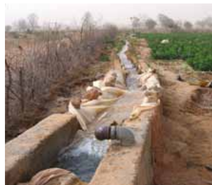
Figure 13: Canal erosion at motorized pump outlet
