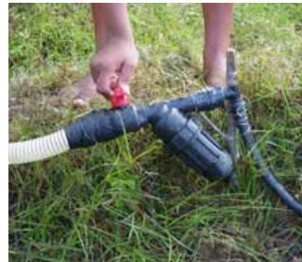
Figure 19 (left): Installation of drip irrigation lines
